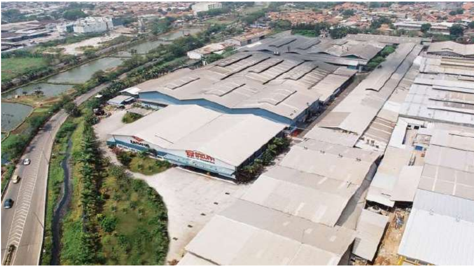
Kapuk Plant (Radiator Facilities)
